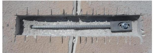
**Step E:** Using a ratchet and 3/4" socket, tighten the nut on the anchor approximately 3-4 turns up to 50 Ft-Lb torque. Locate each stitch carefully. Mechanical Stitch installation is designed for permanent placement. Once installed and tightened down, the anchor cannot be easily removed or relocated.
